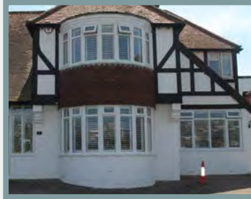
Projected bowed bay with casement windows
