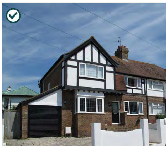
Figure 79: An example of smaller side extension, with matching building materials and colours, to harmonise with the original building, Linchmere Avenue.
