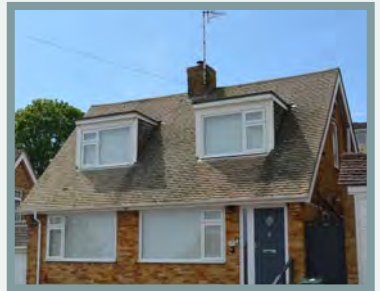
Brown plain tiled gable roof with symmetrical shed dormers
