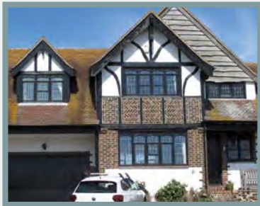
Mock Tudor half-timbering and herringbone brickwork
