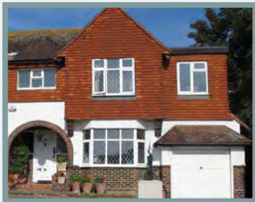
Red hung clay tiles, brick plinth, brick cornices and detailing
